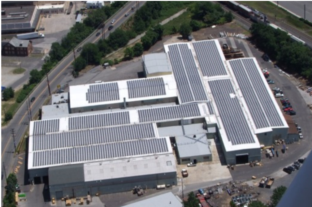
Aerial view of the 4,790 MAGE POWERTEC PLUS modules on the Pennsauken Plant of Philadelphia Sign Company. © Philadelphia Sign Company 2011
